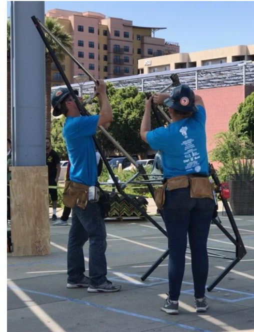
Figure 15: Construction at 2018 PSWC Photo By: Dionne Parrish
