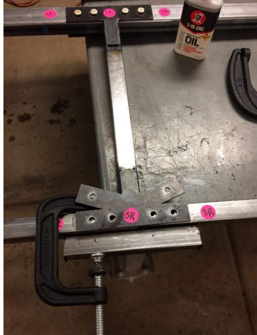
Figure 12: Preparing for Drilling Bolt-Holes Photo By: Isaac Block
