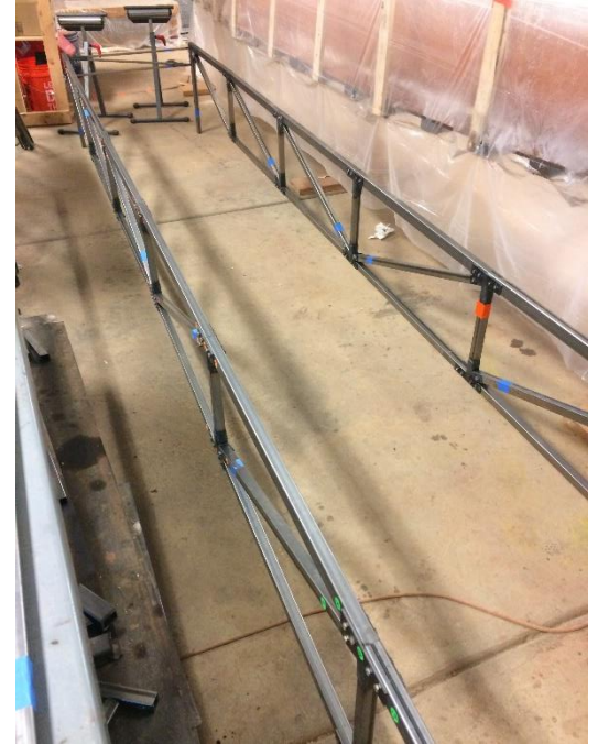
Figure 13: Completed Trusses and Footings Photo By: Isaac Block
