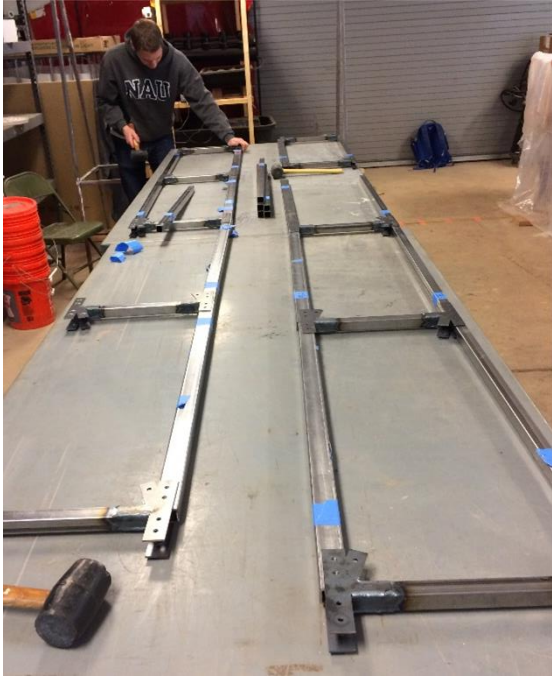
Figure 11: Lining Up Truss Members Photo By: Isaac Block
